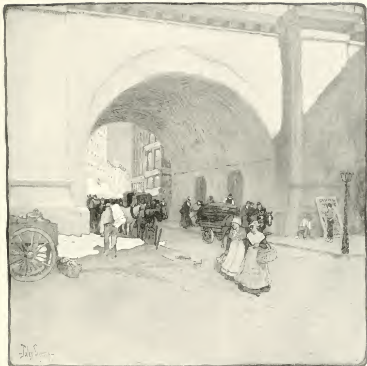
Under the Approach to Brooklyn Bridge.
